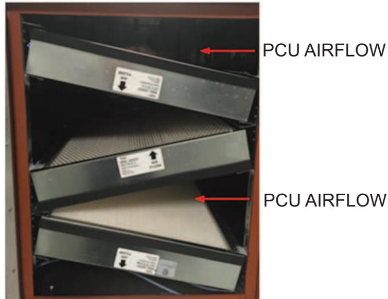
**NOTE: Filters installed with directional arrow stickers match the direction arrows on the PCU frame.**
