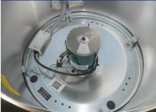
PHOTO 3 Direct-Drive Exhaust Fan. No belt can fail and cause heat/smoke issues. Also no belt drive losses and belt maintenance required.
