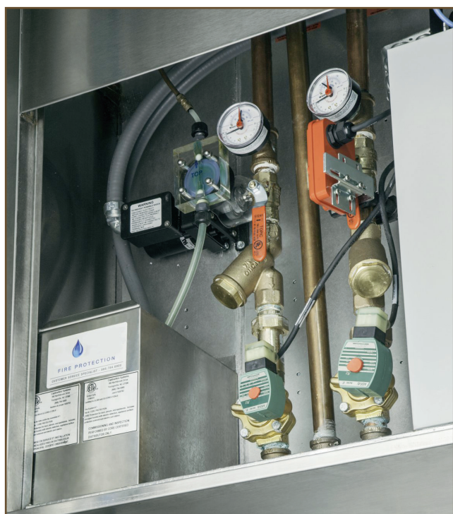
Figure 5. Electronically operated fire suppression system, showing surfactant tank and pump, along with hot and cold water pipes, valves and gauges
