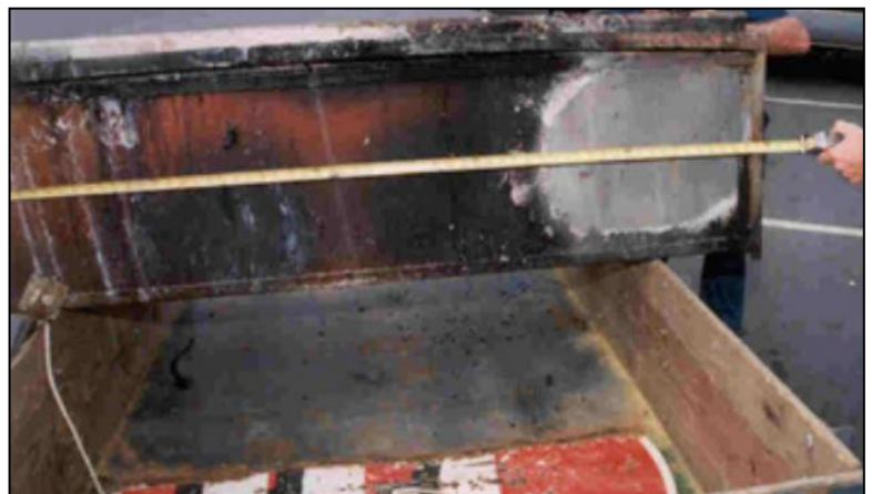
Figure 2. View of the back of the cheese melter with heat pattern on the right corresponding to the origin area on wall.
