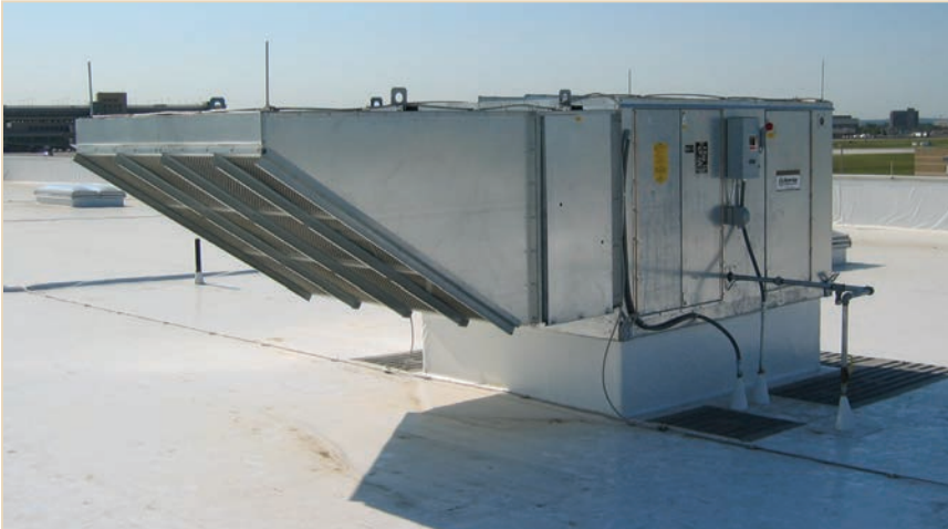
PHOTOS 1 AND 2 Examples of horizontal rooftop and vertical ground-mounted direct-fired units.
