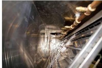
Water mist provides another fire suppression function: as the liquid water droplets absorb heat from the fire and vaporize, the water vapor volume produced is more than 1000 times the volume of the liquid water supplied. This huge increase in water vapor volume displaces air and the oxygen it contains, further suppressing combustion. Water droplets that deposit on surfaces coated with grease or creosote will limit surface temperatures to 212 F to rapidly extinguish active combustion.
