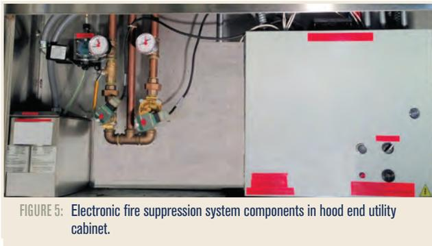
FIGURE 5: Electronic fire suppression system components in hood end utility cabinet.
