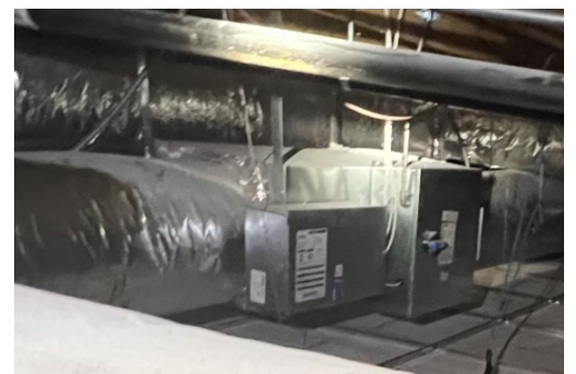
Figure 2 - MZVAV Box - one per zone
