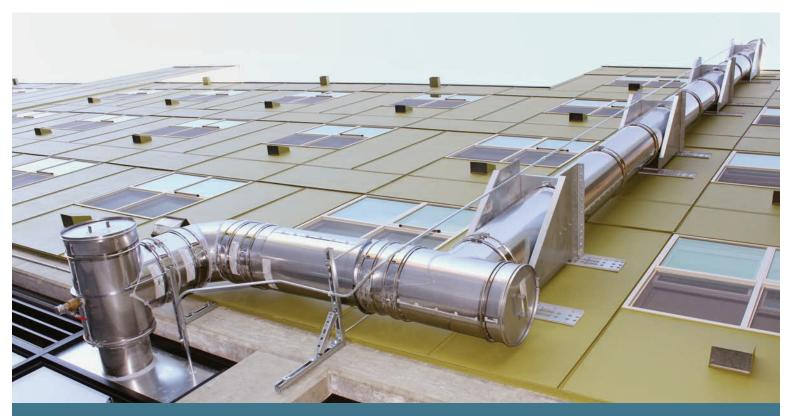
DOUBLE WALL GREASE DUCT
